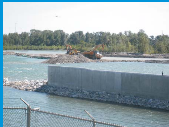
Looking south at the constructed wall extension Completed spring 2009
