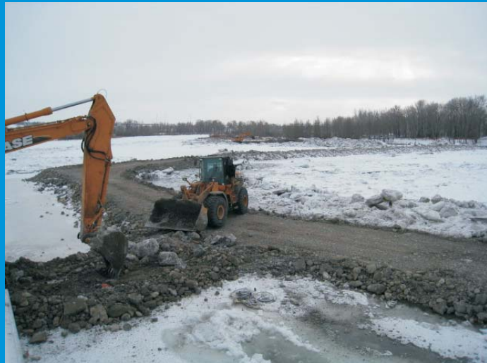
Contractor's cofferdam construction winter 2008
