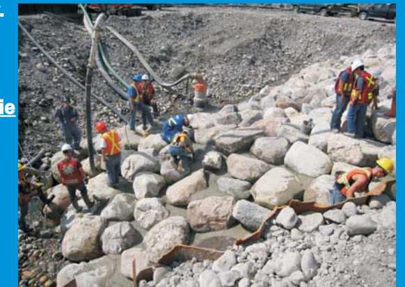
Boulder concrete work on low water channel (river right)
